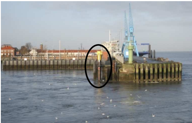
Fig. 1: Location of the Pile/Platform at the north Side of the Entrance of Amerikahafen at Steubenhöft
