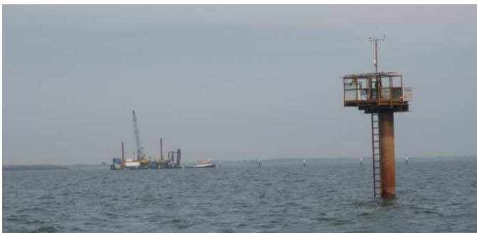
Fig. 2: Offshore-Platform south-east of Borkum
